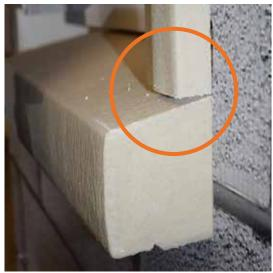
Fit to sill top first - hold moulding to sill and note the sill edge gap
