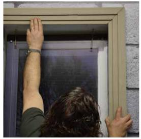
Fit in place using low expansion foam and gun and check levels
