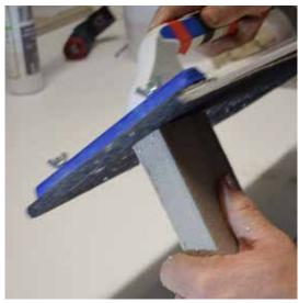
Scribe cut straight edge and sand to fit, continuing to check against sill top
