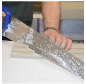
Cut mitred edge with wide toothed saw and double check against reveal
